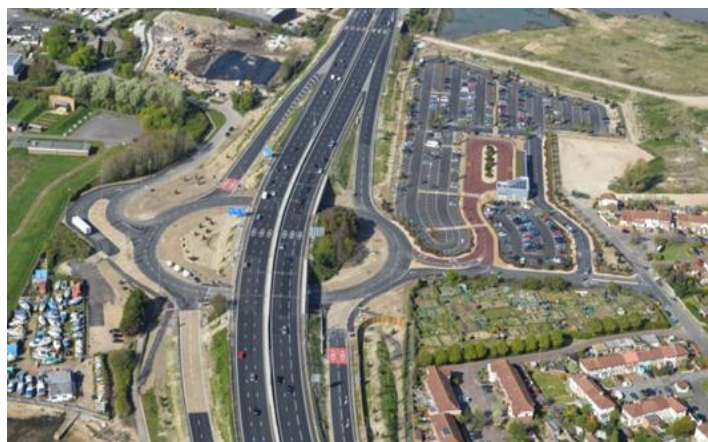
M275 junction and Park & Ride site
